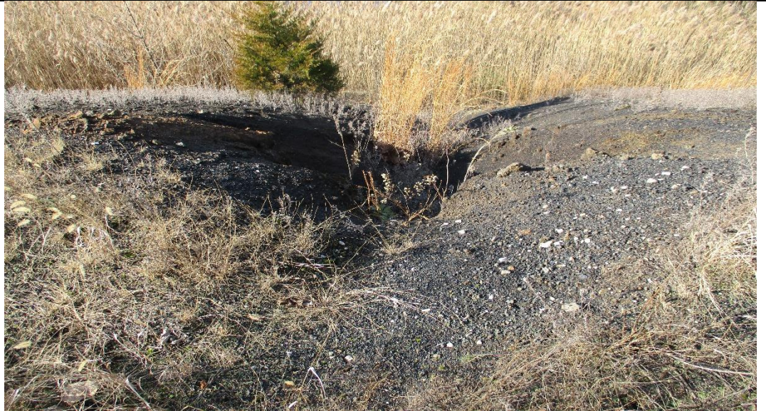
Photograph No. 10 Typical erosion gully.
