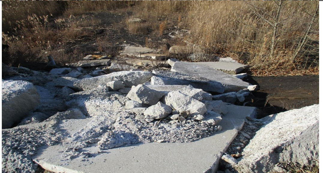
Photograph No. 11 Concrete debris dumped.
