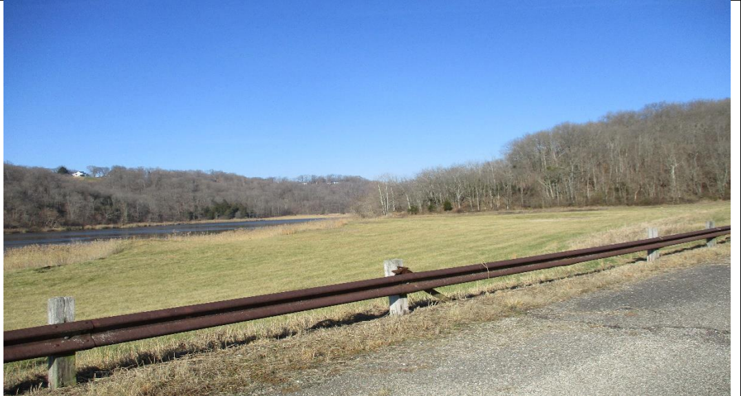
Photograph No. 23 The crest and upstream slope (looking northeast).
