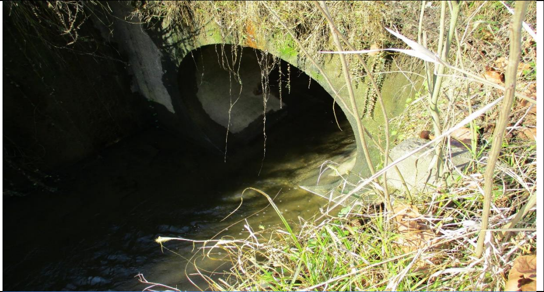
Photograph No. 22 Outfall pipe.
